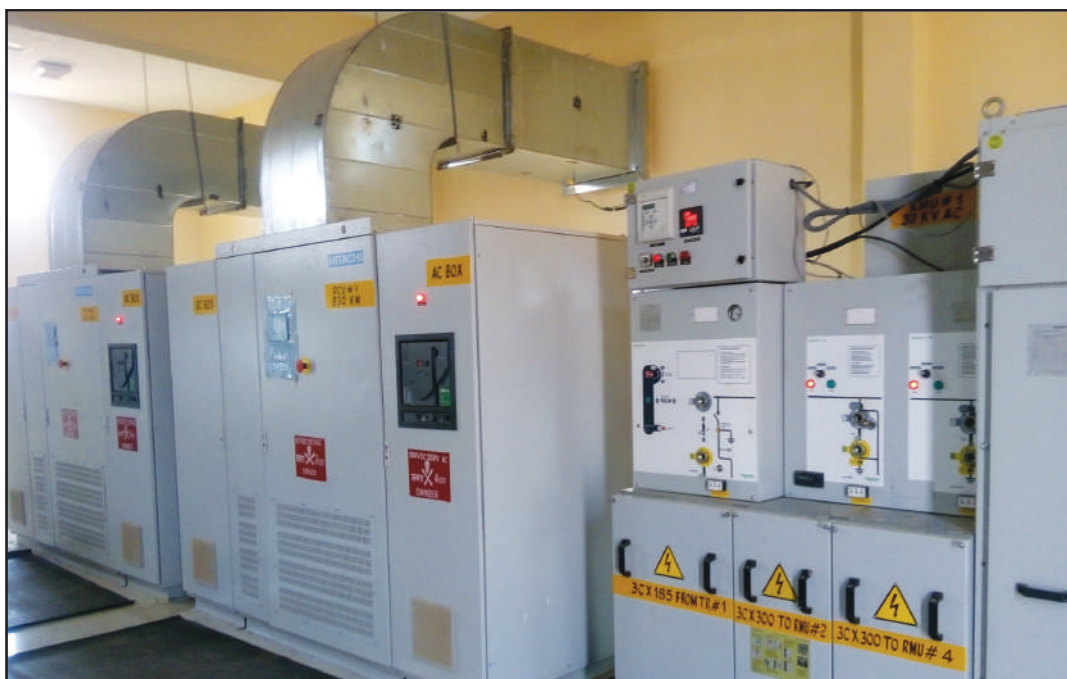
SPP Inverter Room of 20 MW PVSP, Manmunda
