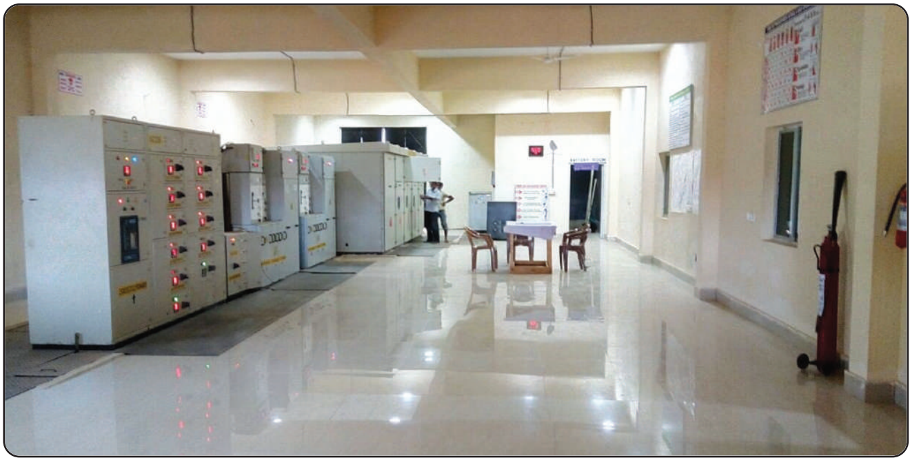
Main Control Room of 20 MW PVSP, Manmunda
